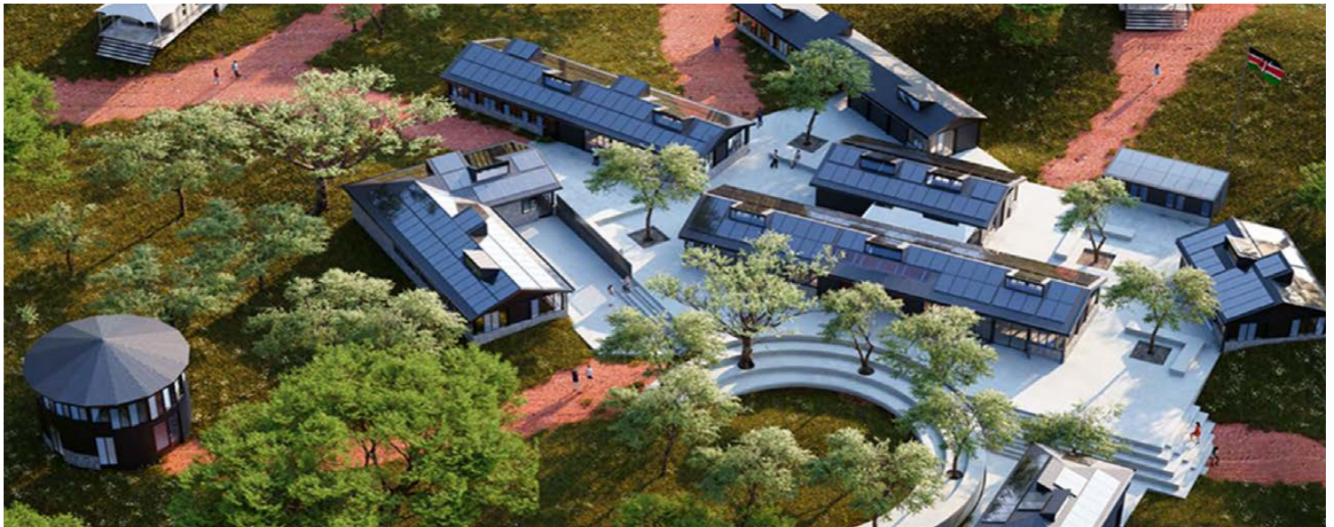
Projects in Pardamat CA included construction of a wild- life dam fed by Koyiaki Natural Spring and construction of the Wildlife Tourism College.
